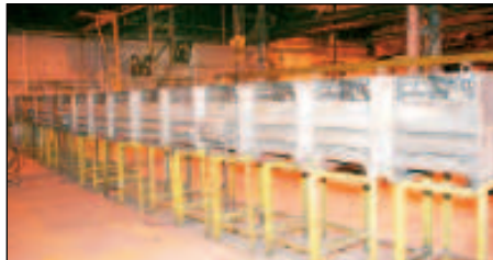
View of Welders
