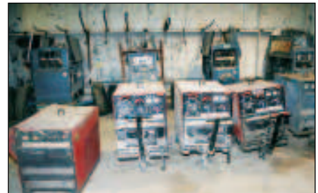
View of Welders
