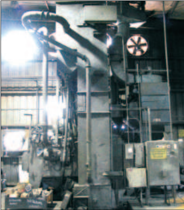
Pangborn Blast Clean System
