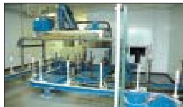
600' Approx. Nutro on Edge Conveyor System
